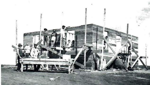
The new house under construction. Built in 1919.
